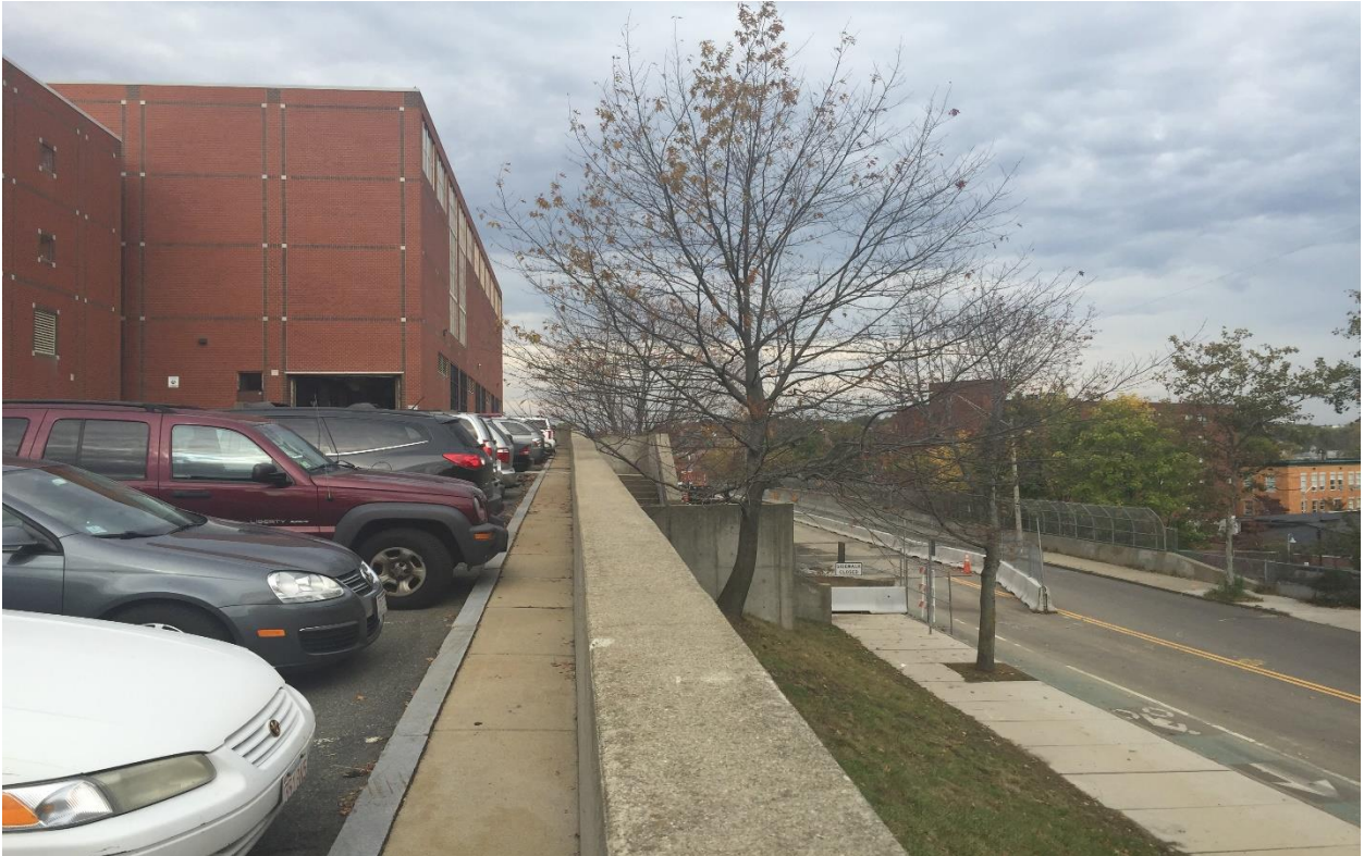
Back of 1988 Wing with View Toward Medford Street
