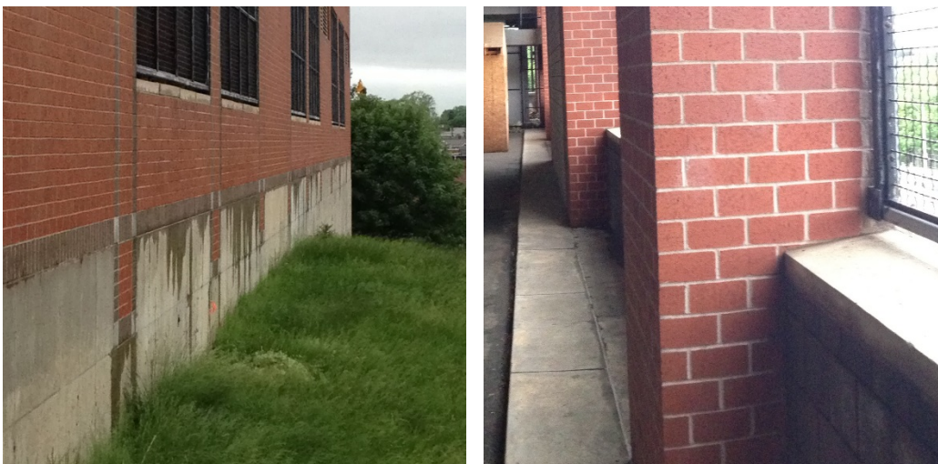
Exposed Concrete Foundation and Brick Connections
