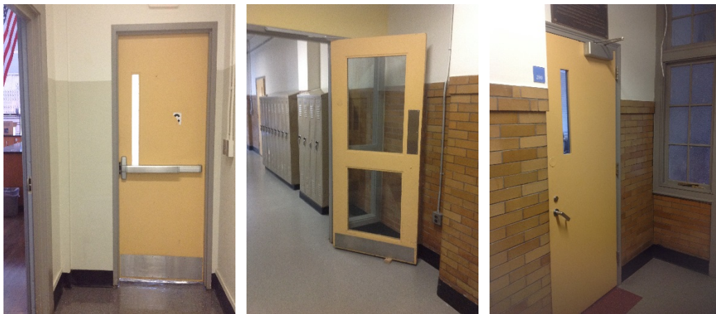
Doors and Door to Stairs
