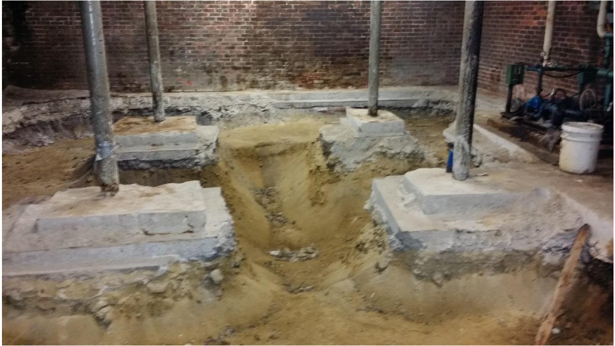
Room off of Boiler Room with Excavation
