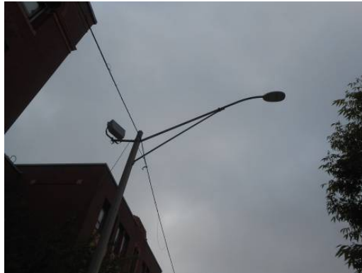
Cobrahead Fixture with Flood Light
