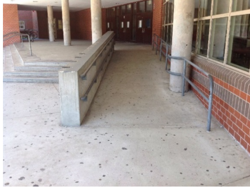
E Wing Ramp
