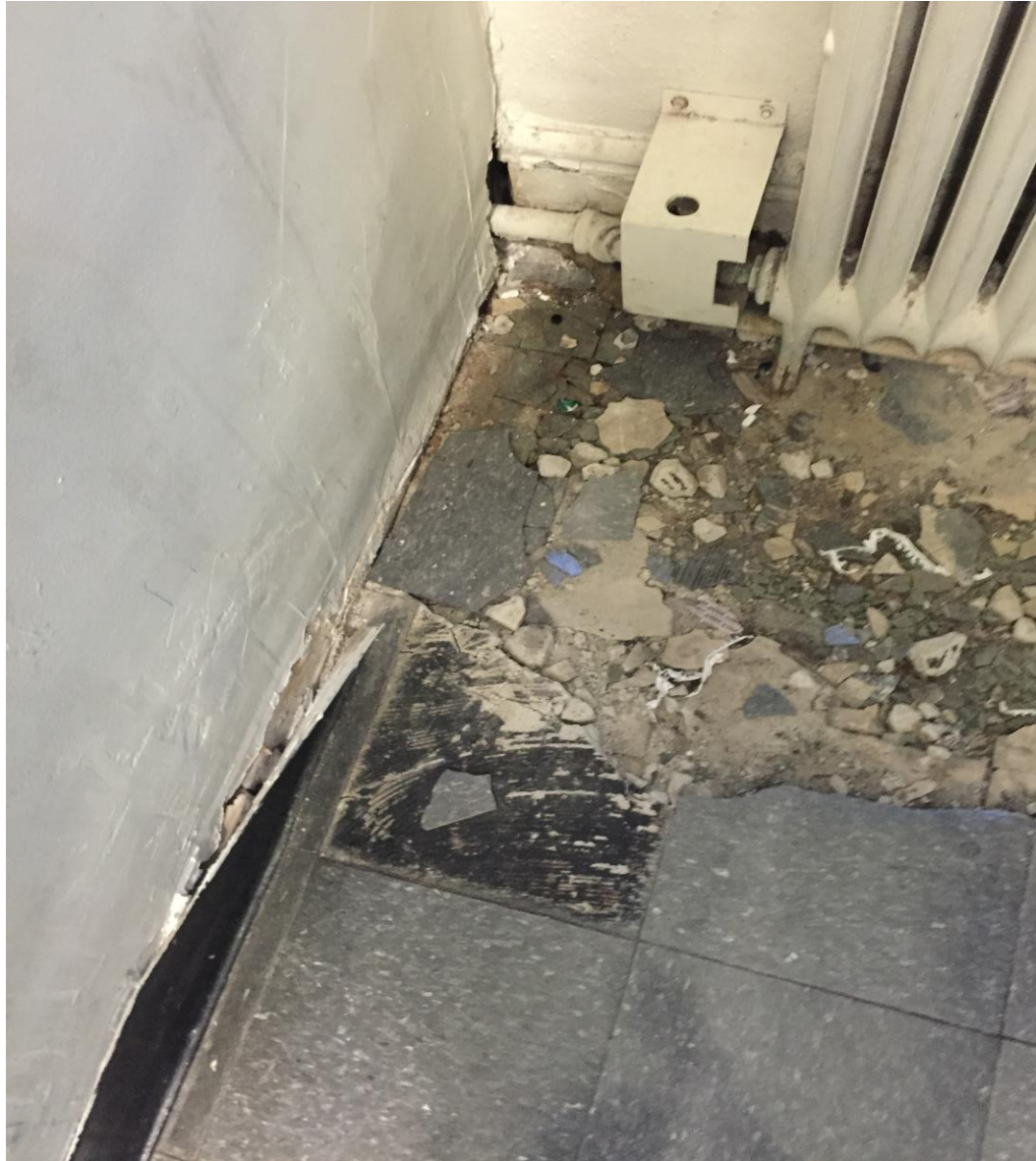
Multiple Layers ACM Flooring B Wing
