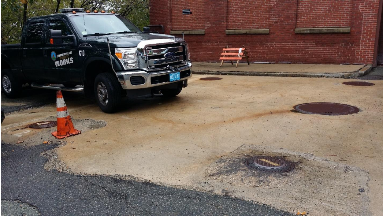
15,000-Gallon Fuel Oil USTs Near Loading Dock
