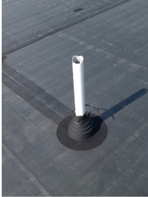
Photo 12: Lab Vent through roof in poor condition
