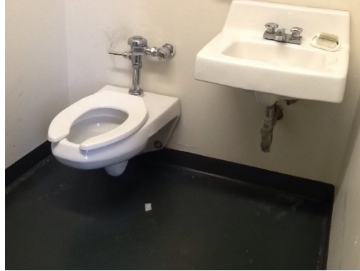
Photo 19: Existing water closets
