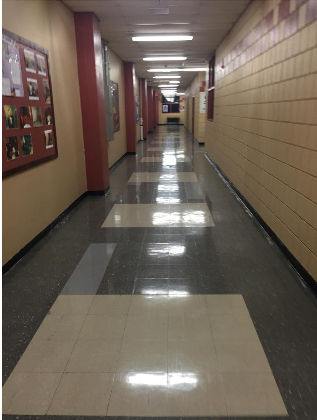
ACM Floor Tile in 1988 Wing
