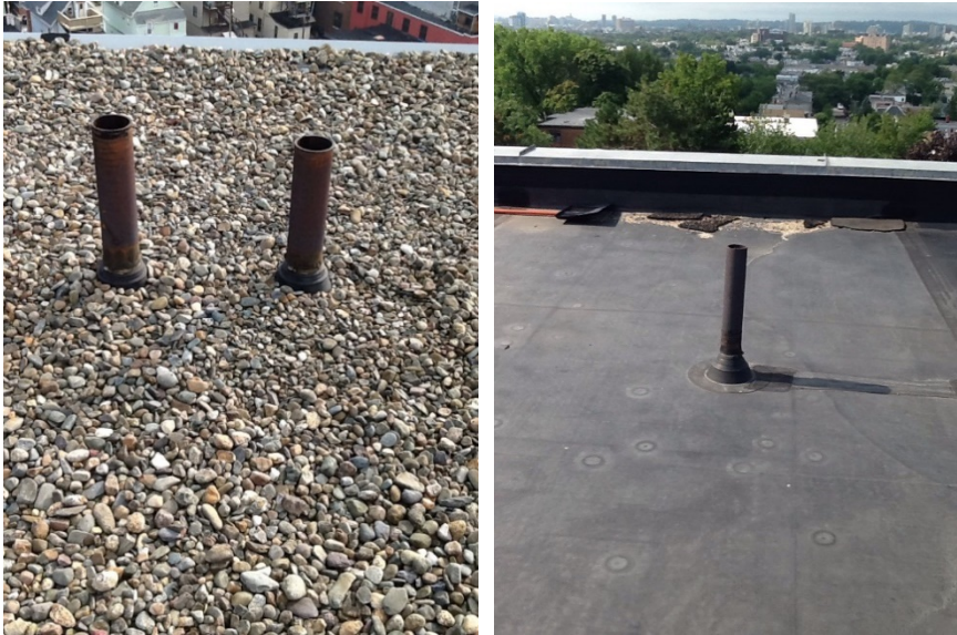
Photo 7: Vents through roof in poor condition
