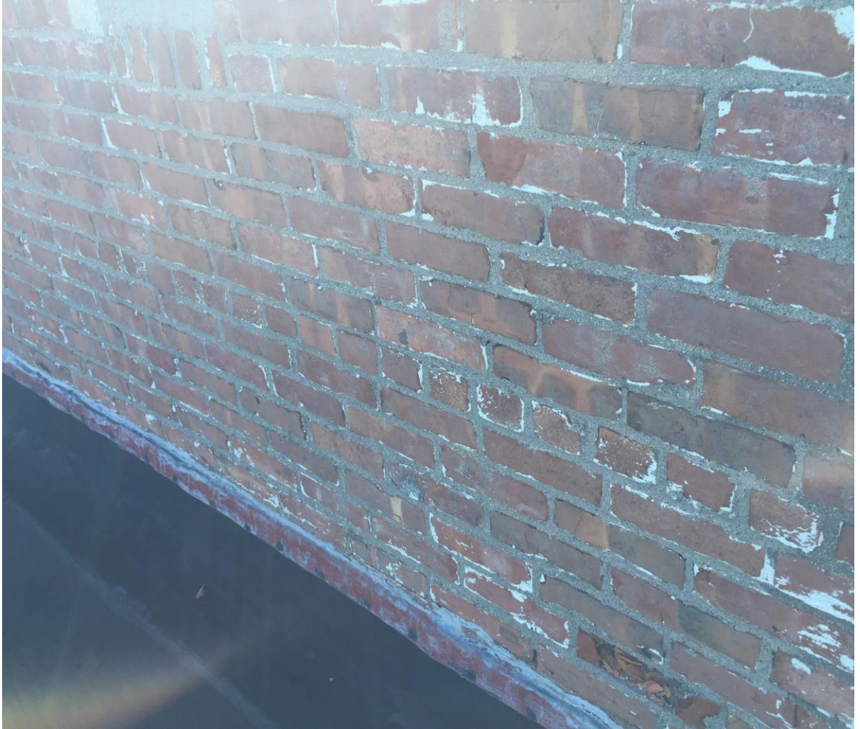
ACM Caulk on B Wing Roof Auditorium
