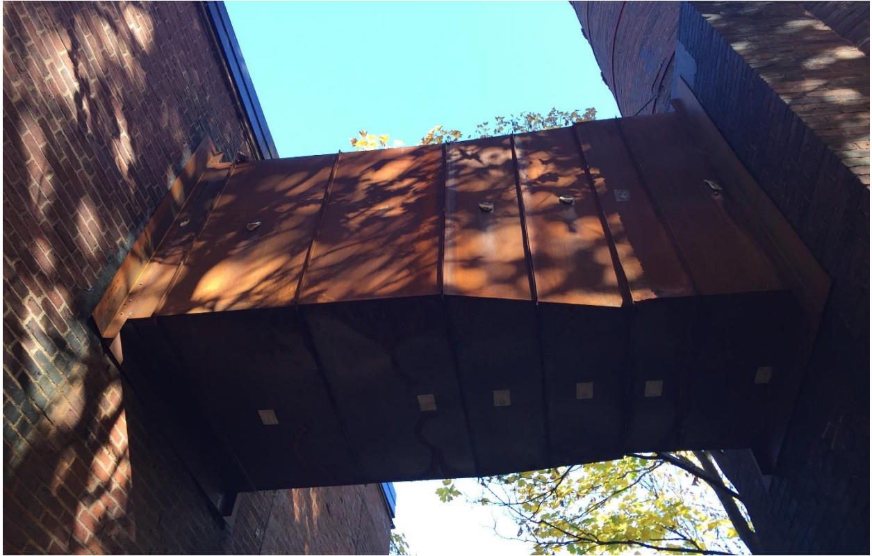
Discharge to Chimney
