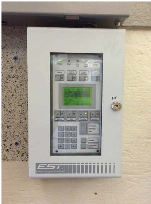
Annunciator for Wing A, B, C
