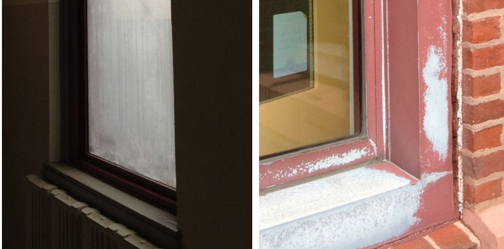
Fading Anodized Aluminum Finish
