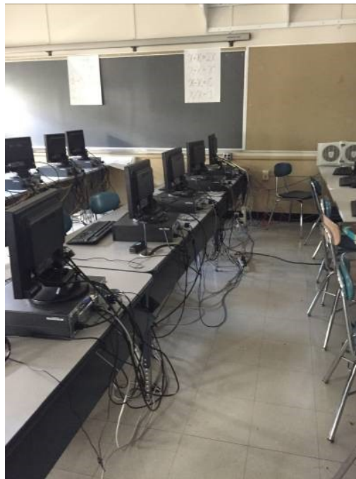
Lack of Receptacles Where Needed
