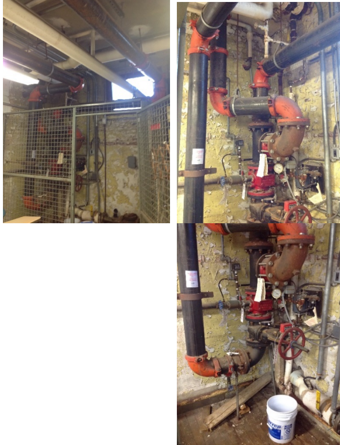
Photo 2: Existing Fire Service
