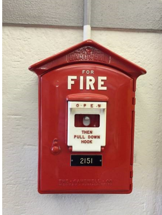
Master Box for Wing A, B, C
