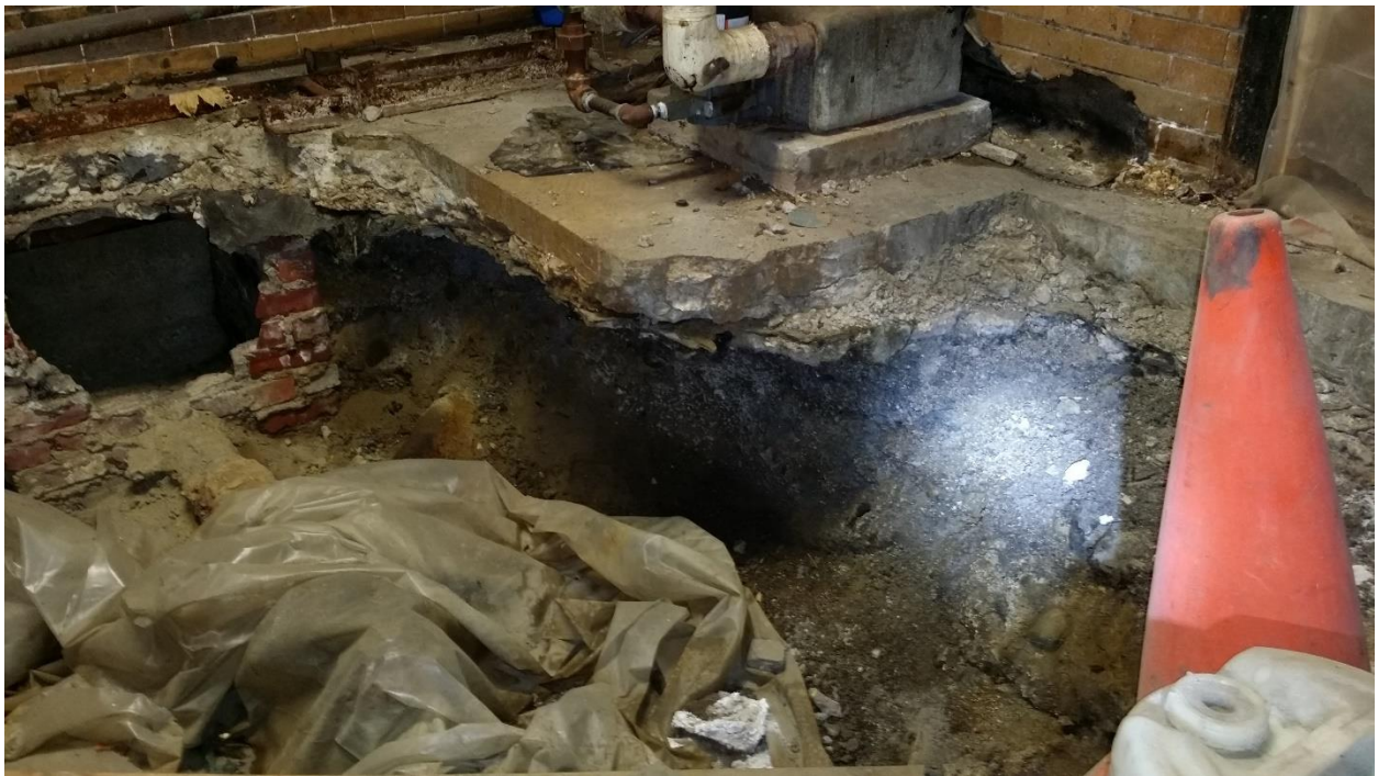
Room off of Boiler Room with Excavation
