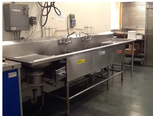
Photo 10: Waste Piping Installation at Triple Pot Sink
