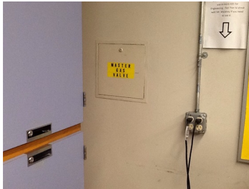
Photo 5: Not accessible emergency gas shut-off valve
