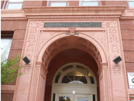
Building Sign Lighting
